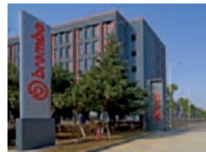
Nanjing integrated industrial hub (China).
